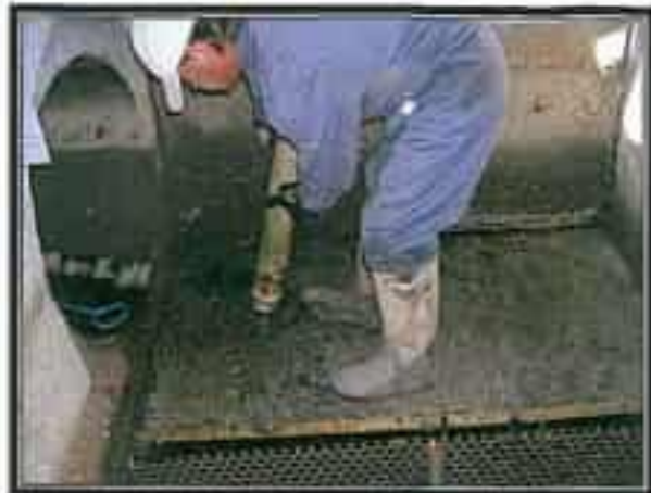
Picture No. 16: Unit #1 Influent Screen Cleaning
