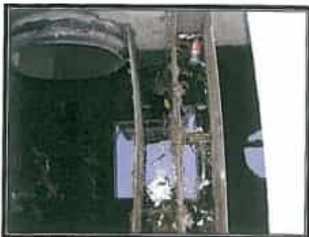
Picture No. 9: Unit #2 Influent Compartment, Weir Screen and Oil/Water Separator
