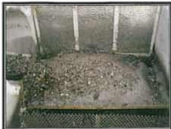
Picture No. 3: Unit #1 Influent Screen Sedimentation after flushing event storm (front screen removed)
