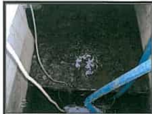
Picture No. 6: Unit #1 Influent Screen heavy leaf litter
