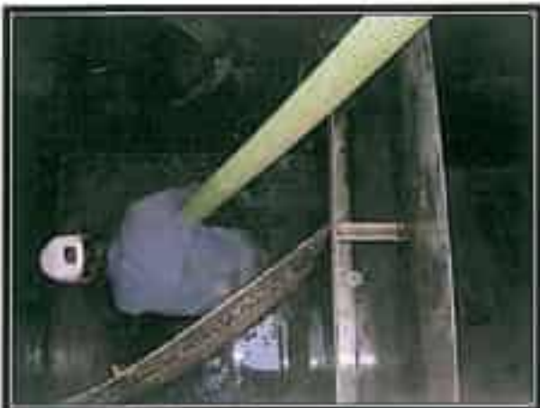
Picture No. 17: Unit #2 Vacuum Cleaning
