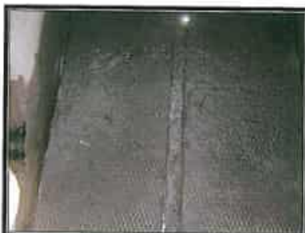
Picture No. 12: Unit #2 Filter Fabric Screen caked with typical sludge
