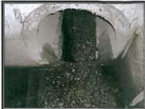
Picture No. 4: Unit #1 Influent Pipe Sedimentation
