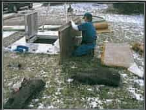
Picture No. 18: Unit #2 Filter Fabric Replacement
