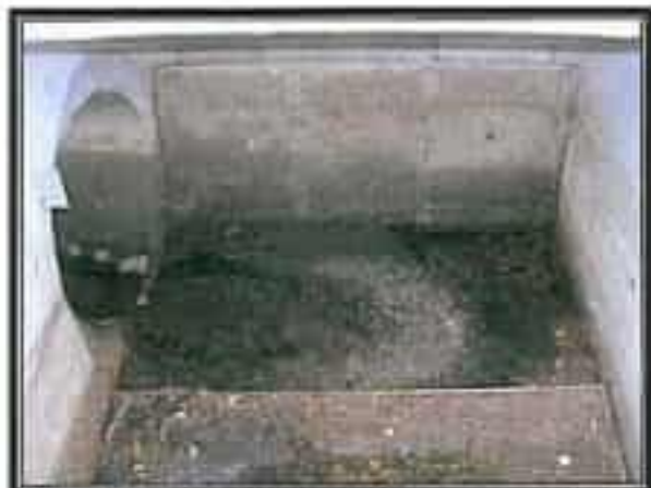
Picture No. 5: Unit #1 Influent Screen typical debris and sediment (front screen shown down)
