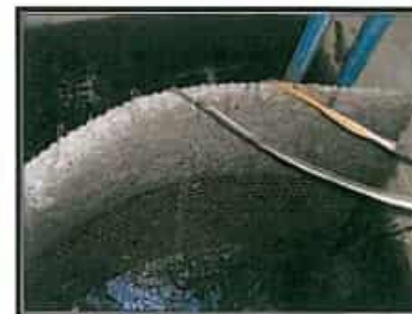
Picture No. 8: Unit #1 Weir Screen top blinded
