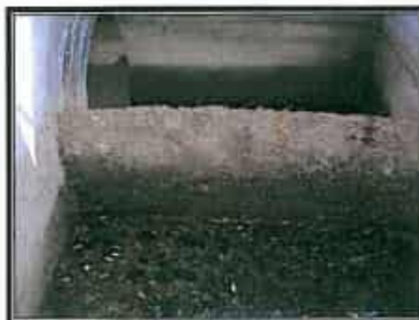
Picture No. 7: Unit #1 Weir Screen retaining floatables
