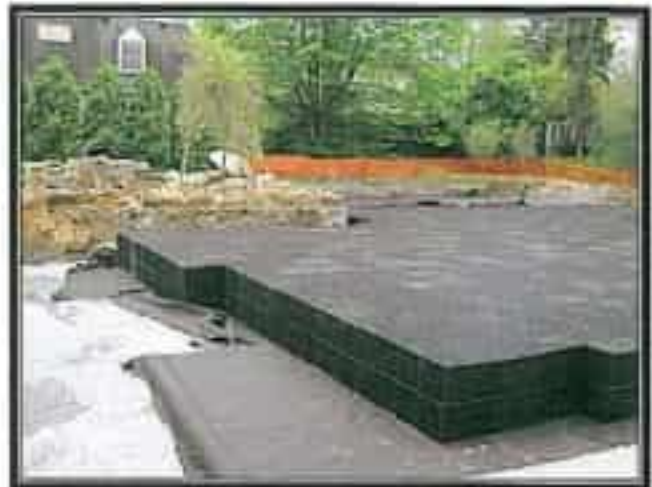
Picture 2: RainTank® Assembly Installation
