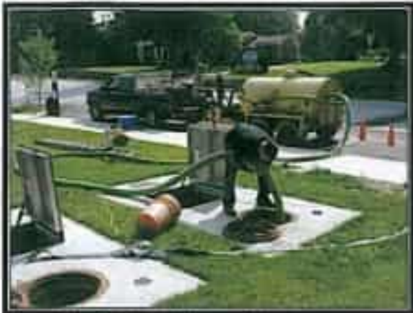
Picture No. 15: Unit #1 Vacuum Cleaning
